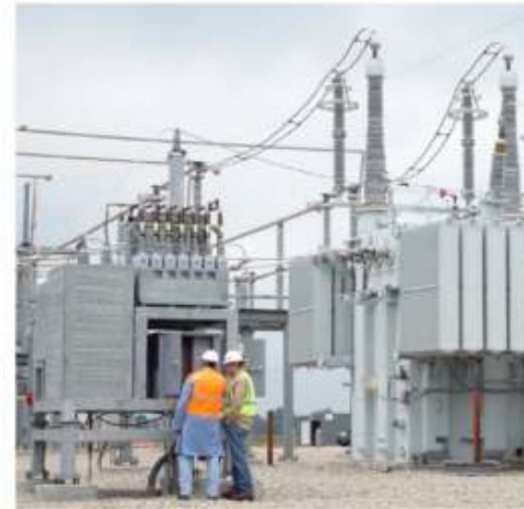
GIC Blocking Device Connected to Large Power Transformer RELIABILITY | RESILIENCE | SECURITY
