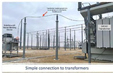
This prevention of half-cycle saturation removes the heating, VAR consumption and harmonic effects
