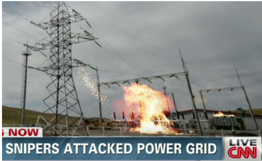
Screenshot from CNN reporting on 2013 sniper attack on PG&E's Metcalf transformer station in California.
