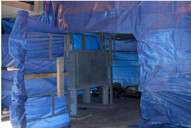
Figure 7: Temporary windbreak created with scaffolding and tarpaulin
