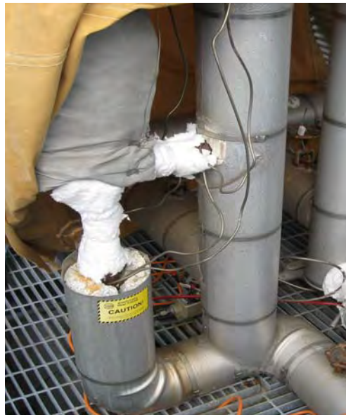
Figure 4: Insulated Piping with Heat Tracing
