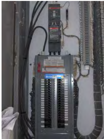
Figure 1: Freeze Protection Panel Interior
