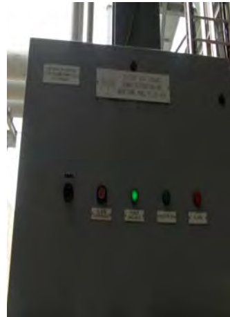
Figure 2: Freeze Protection Panel Exterior
