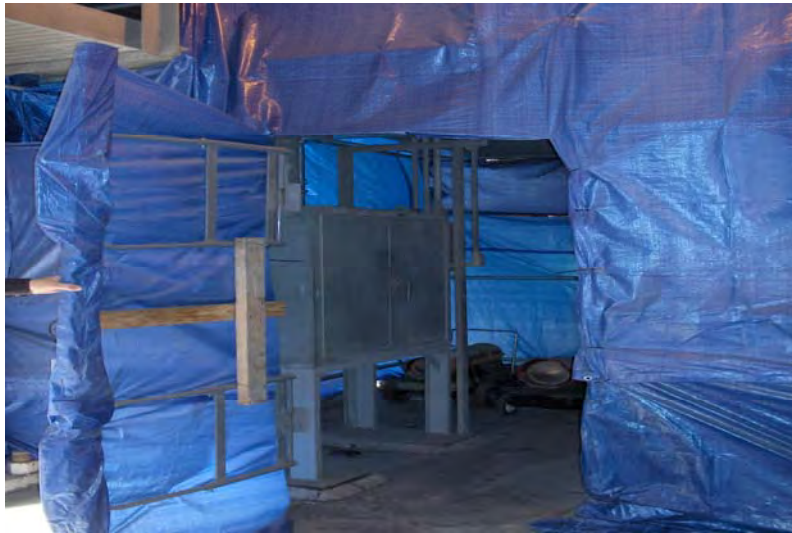
Figure 7: Temporary windbreak created with scaffolding and tarpaulin
