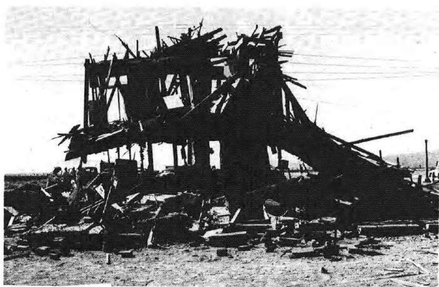
Figure 5.67. Unreinforced brick house after a nuclear explosion (5 psi peak overpressure).
