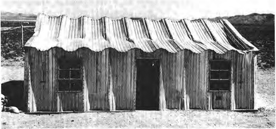
Figure 5.44. Self-framing corrugated steel panel building after a nuclear explosion (3.1 psi peak overpressure).
