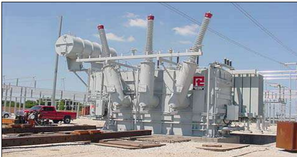
Figure 3. Installation of a 345 kV Transformer
