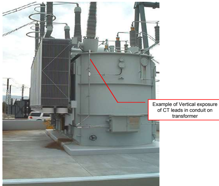
Figure 5-9. Exposure of cable conduits on transformers
