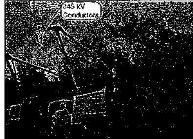
Figure 4.10. Cause of the Hanna-Juniper Line Loss
