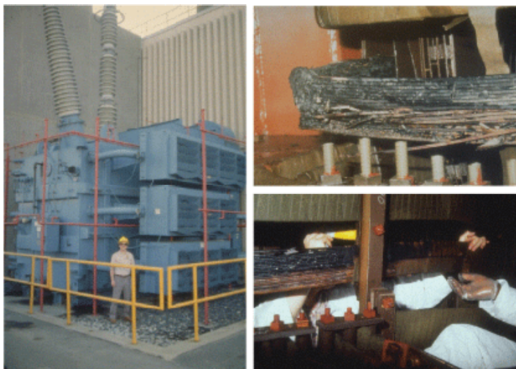
Figure 9: This is a picture of the Salem New Jersey Nuclear Plant GSU Transformer (~1200mVA, 500/22kV single phase transformer) and permanent damage caused by the March 13, 1989 Geomagnetic Storm. Photos courtesy of PSE&G.
