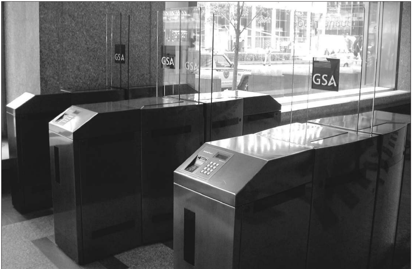
Figure 4: Smart Card Access Portals at the Jacob Javits Federal Building Entrance
