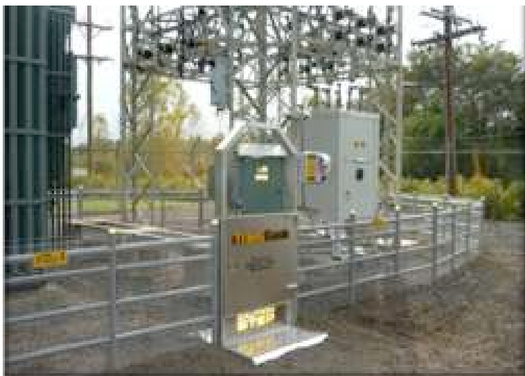
Figure 3.A.5 Electrified Marmot Fence at a Distribution Substation in the Pacific Northwest
