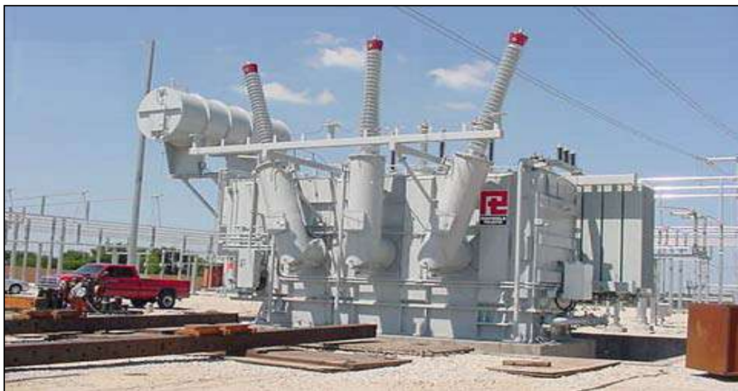
Figure 3. 345 kV Transformer Installation
