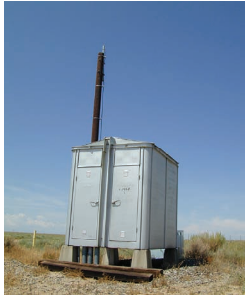
Figure 6-3. Typical Block Signal Control Equipment Enclosure
