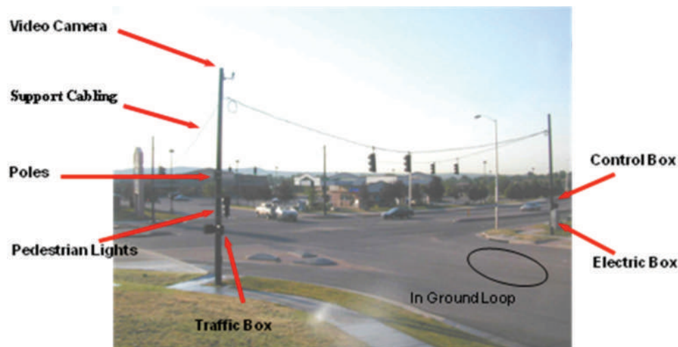
Figure 6-6. A Typical Signalized Intersection
