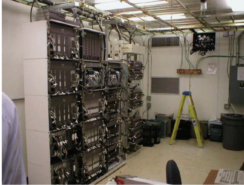
Figure 3-4. Cellular Base Station Equipment
